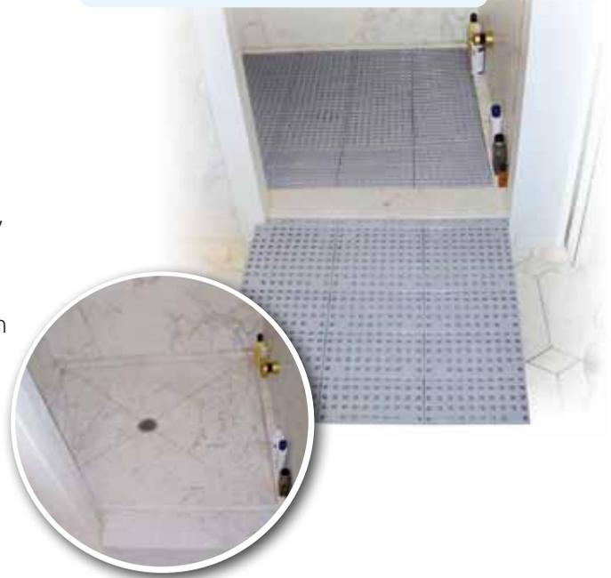
When not enough space is available for a ramp solution, the whole floor should be raised to create optimal accessibility for the user.
